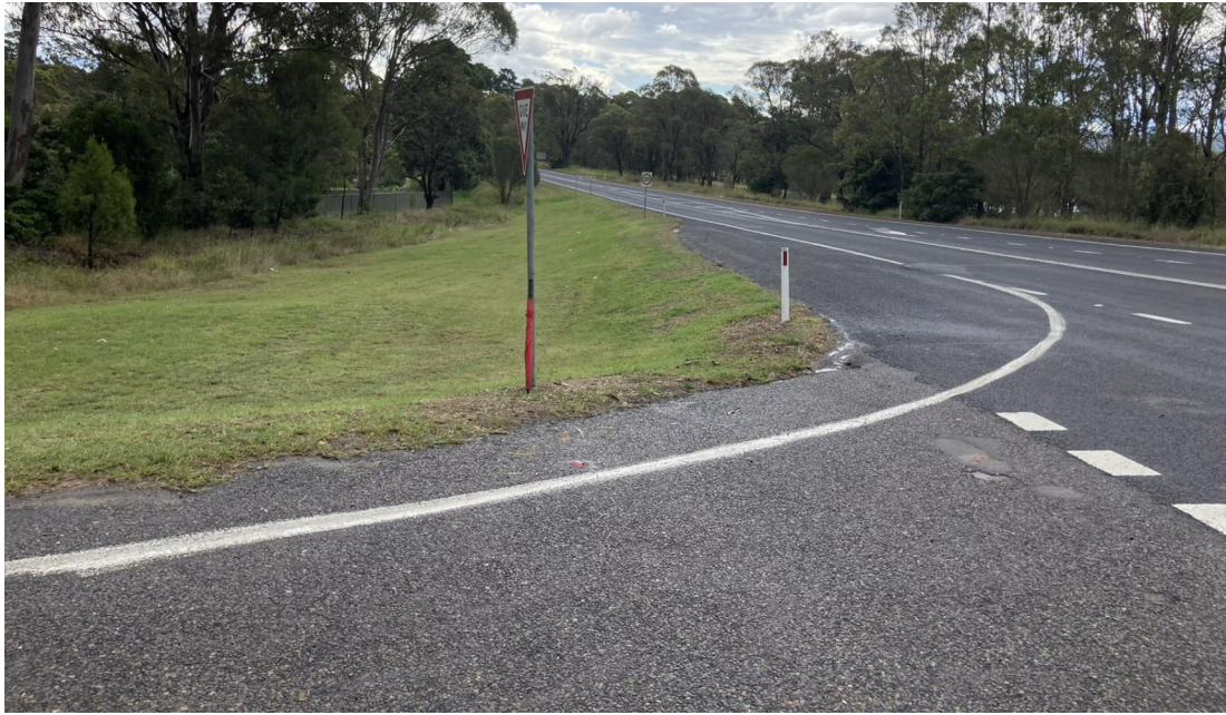
VIEW TO NORTH BEGA ST > PRINCES HWY
