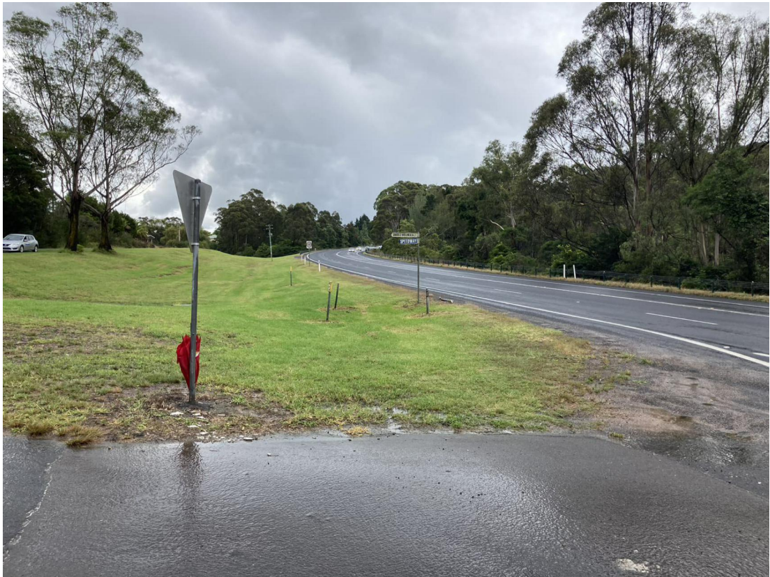
VIEW TO NORTH CANDELO WOLUMLA RD > PRINCES HWY
