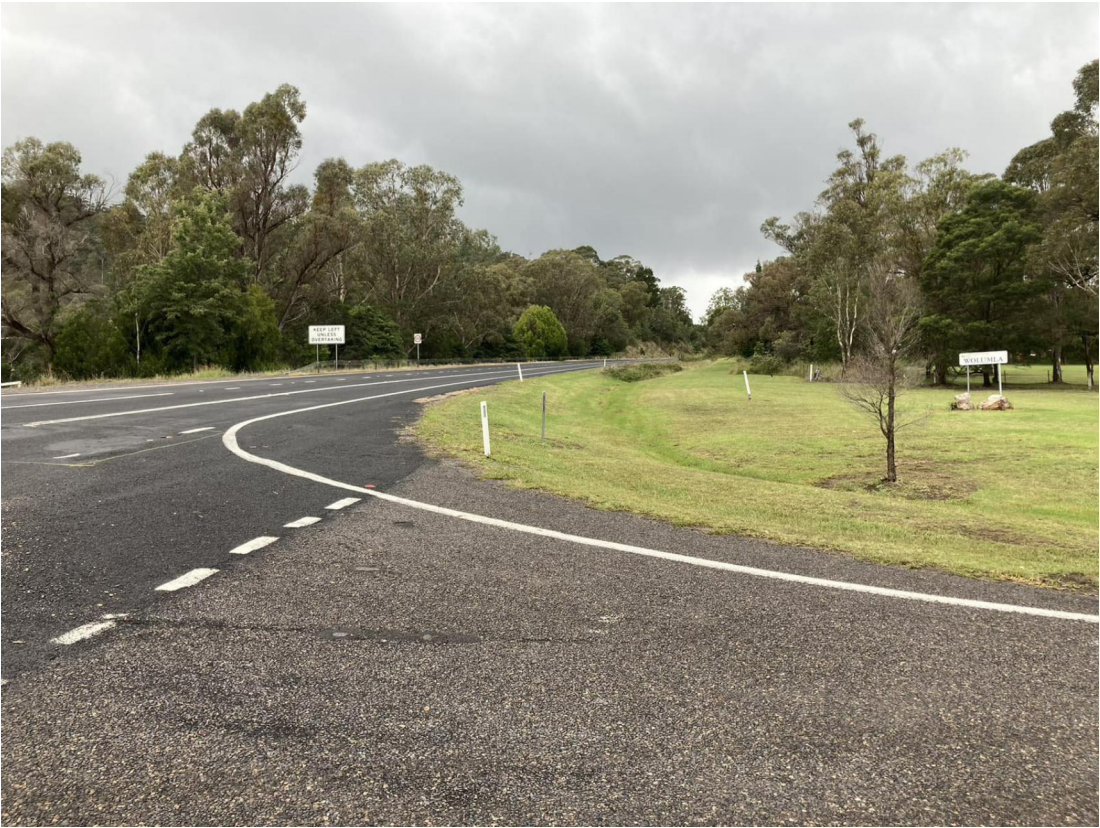
VIEW TO SOUTH BEGA ST > PRINCES HWY
